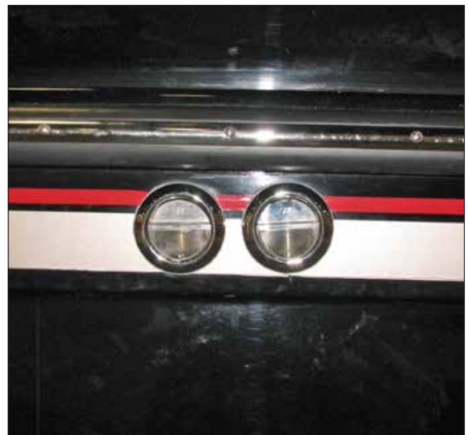
Scupper Drain Thru-Hull Fittings & Check Valves
