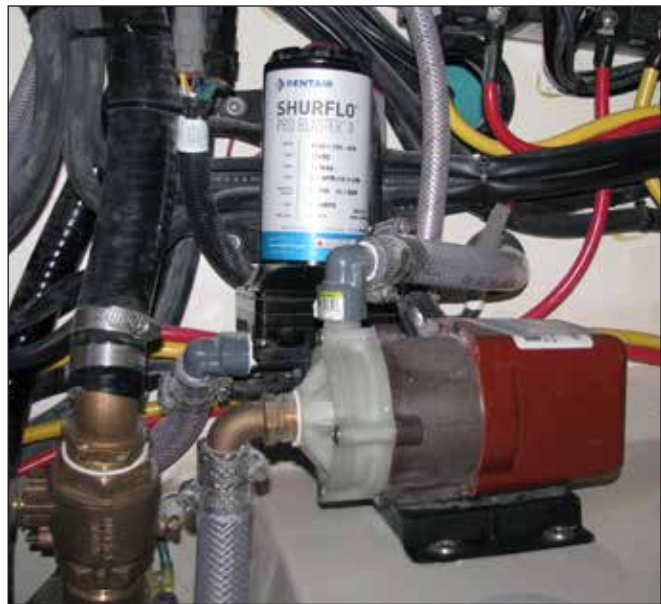
Raw Water Pump & Typical Air Conditioner Or Optional SeaKeeper Cooling Pump
