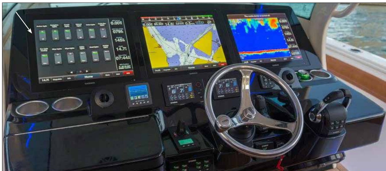
Typical Switch Panel In Helm Electronics Touch Screen Display Panel
