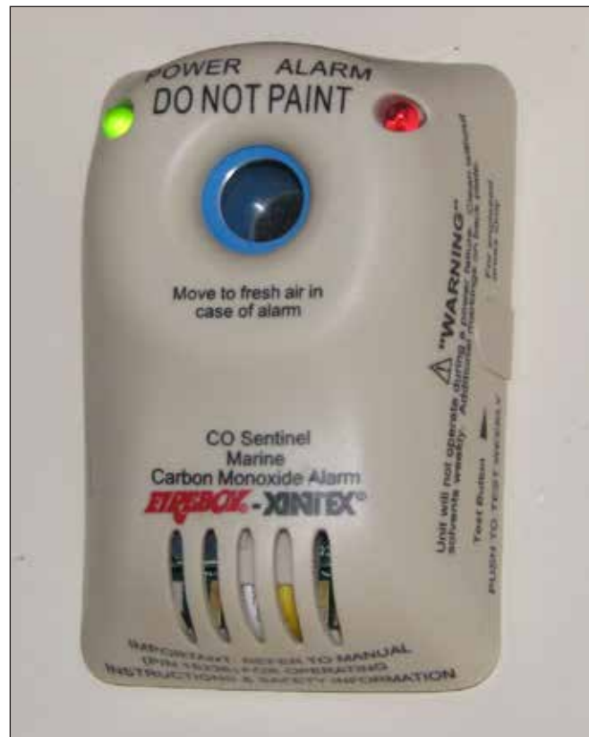
Typical Carbon Monoxide Detector
