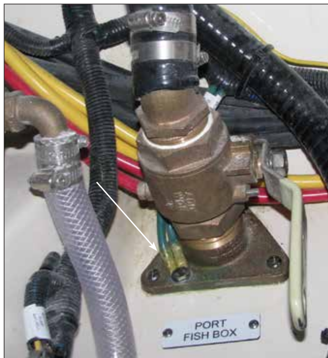
Thru-Hull Valve Bonding Wires & Connection
