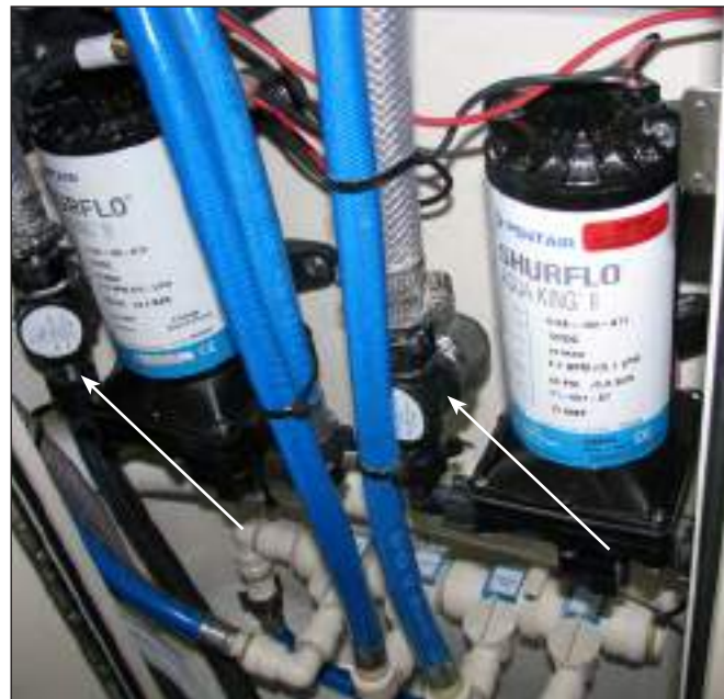
Typical Fresh Water Pump Strainers
