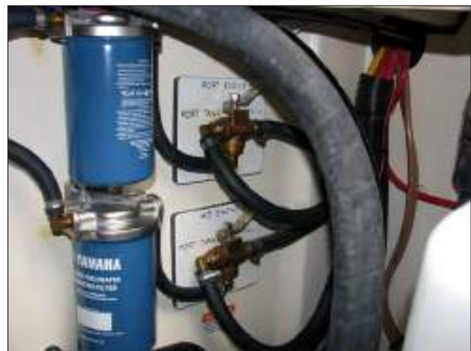
Triple Engine Fuel System - Port & Center Engine Fuel Selector Valves & Filters
