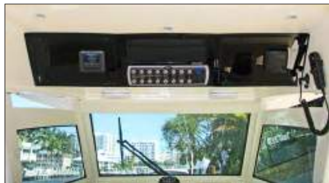
Hardtop Switch Panel & Electronics Above Helm
