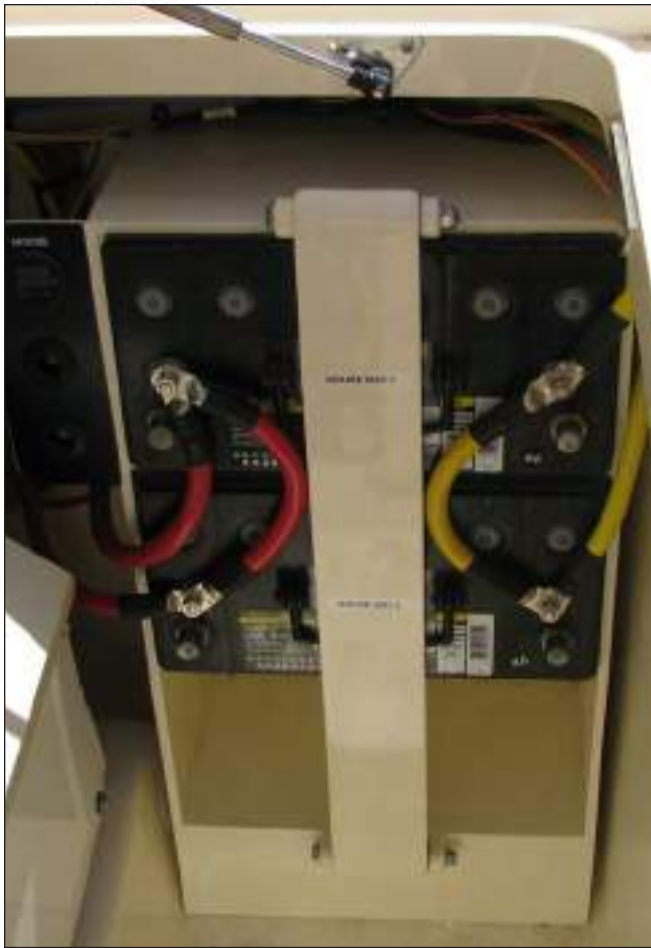
Typical Triple Engine House Batteries
