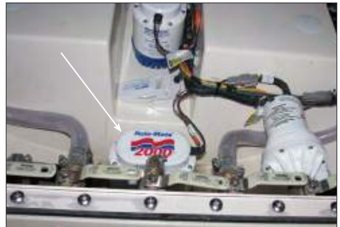
Aft Bilge Pump With Automatic Switch
