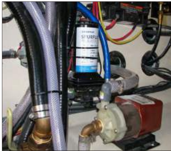
Raw Water Pump & Typical Air Conditioner Or Optional SeaKeeper Cooling Pump
