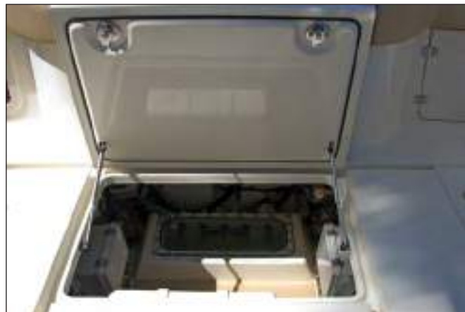
Aft Systems Room Hatch
