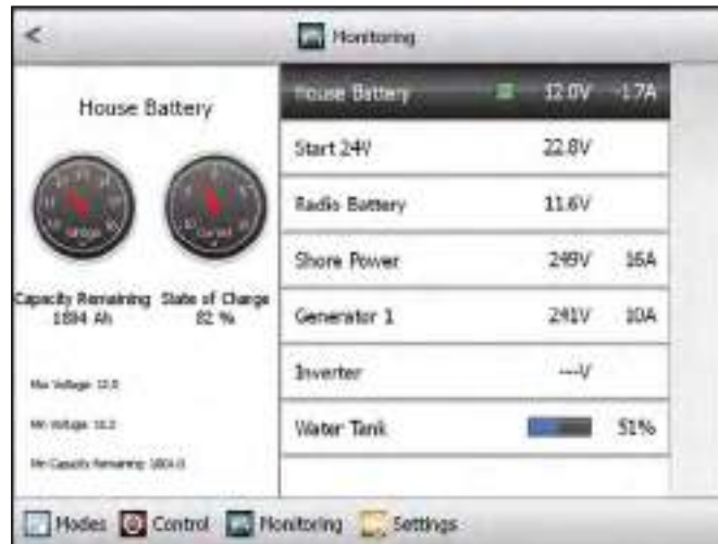
CZone Display Monitoring Screen
