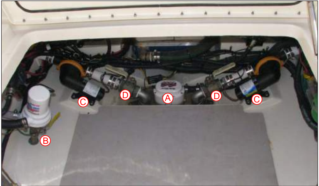
Stern Systems Station and Bilge
