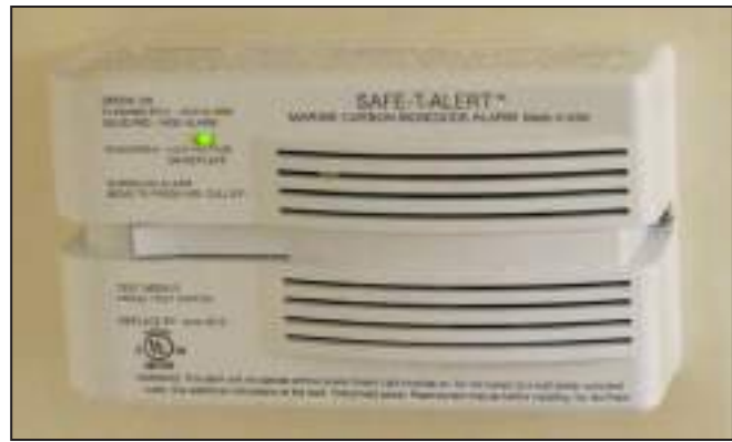
Carbon Monoxide Detector
