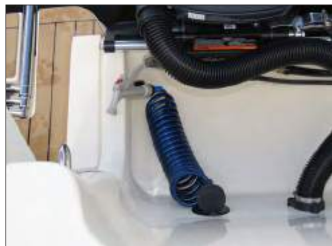
Cockpit Fresh Water Washdown Hose & Connection
