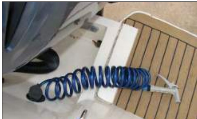
Cockpit Raw Water Washdown Connection
