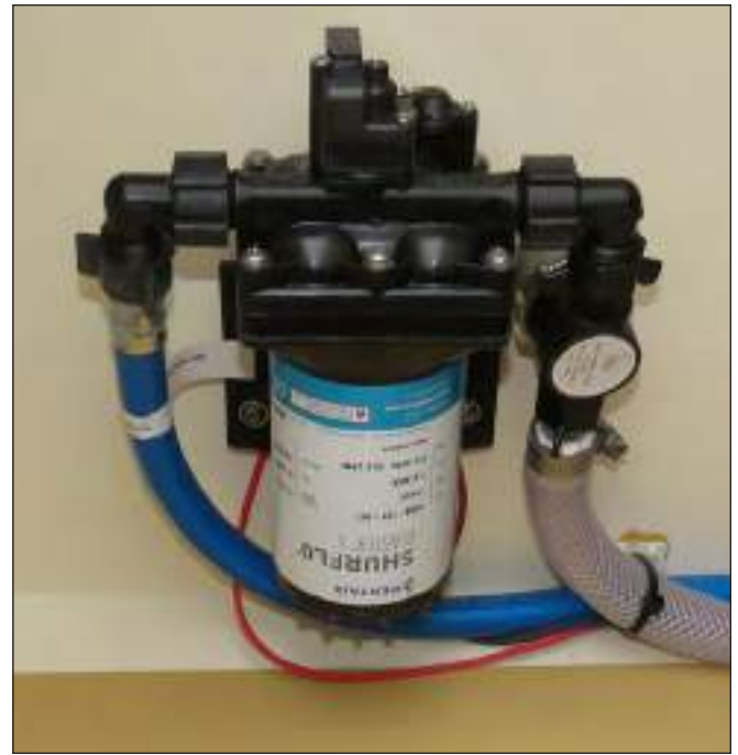
Typical Fresh Water Pump & Strainer
