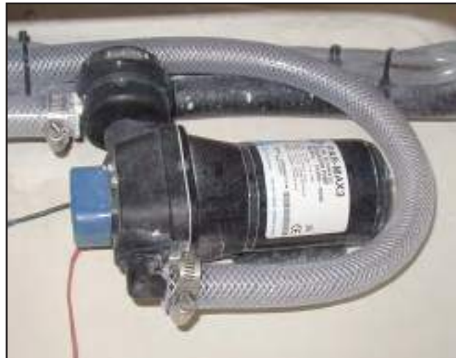
Typical Fresh Water Pump & Strainer
