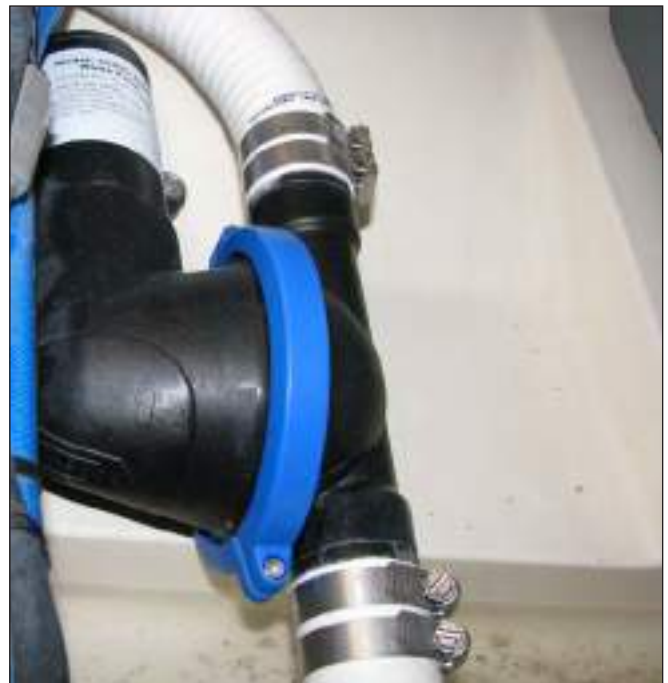
Typical Waste Discharge Diaphragm Pump
