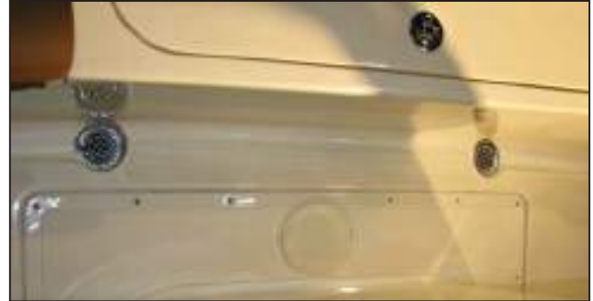
Scupper Drains & Drain Rails
