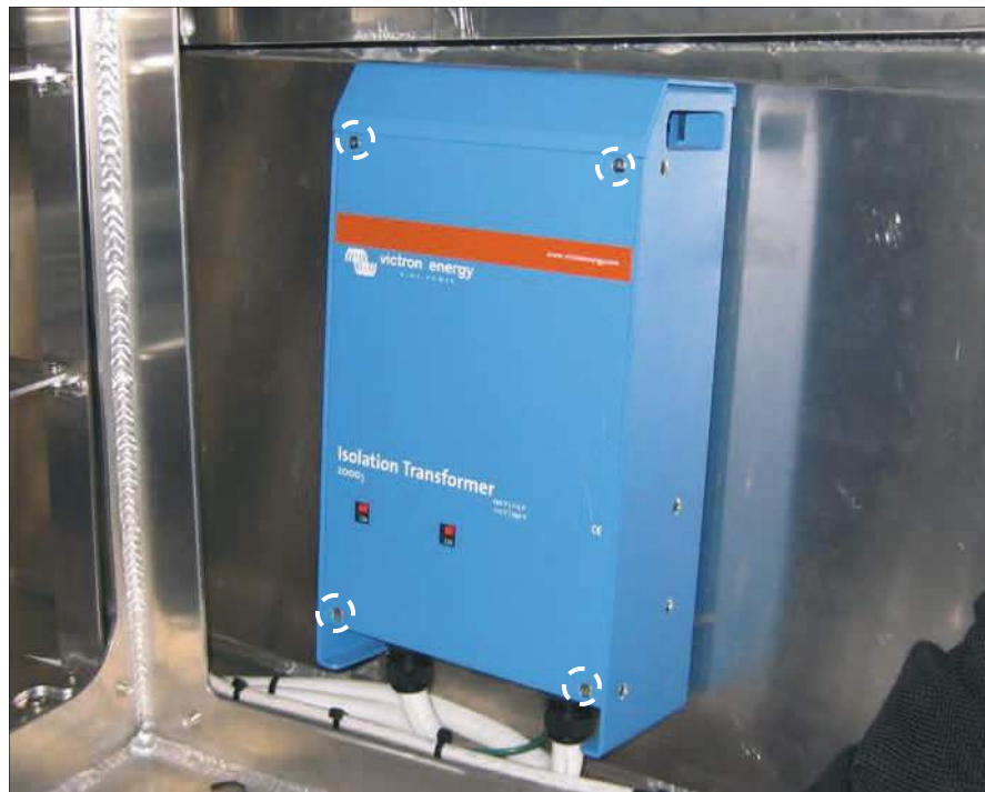
Figure 311-4.1a. Isolation Transformer Cover Plate Screws
