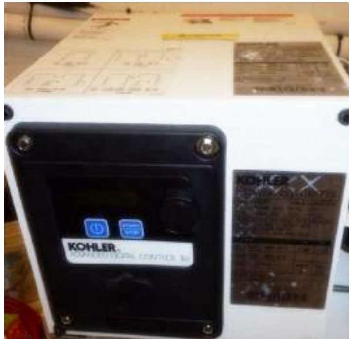
TYPICAL GEN-SET REMOTE ELECTRICAL PANEL
