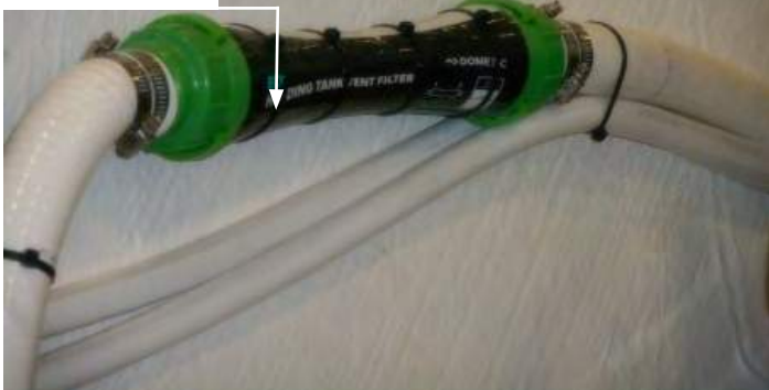
Typical Waste System In-Line Filter
