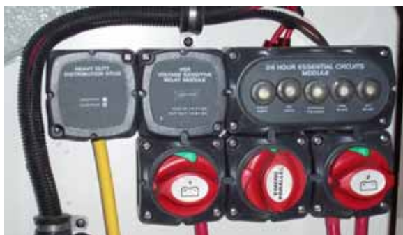
Battery Switches and Main Breakers Single Engines (typical)
