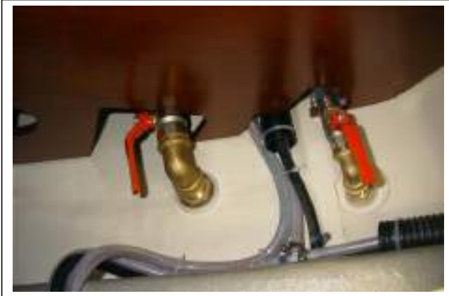
ABB.: RAPID SHUT OFF VALVE – WET AREA
