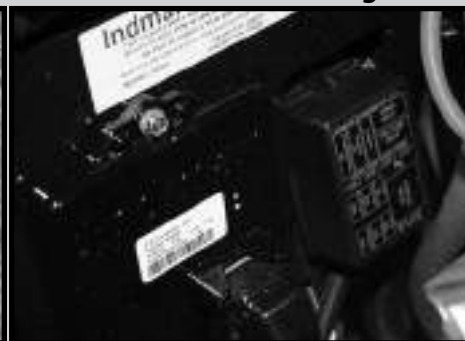
Fuse Panel - Back of Engine
