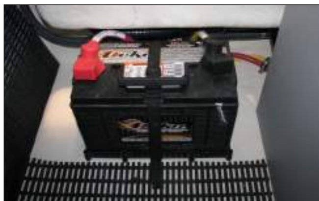
268SS Battery Installation
