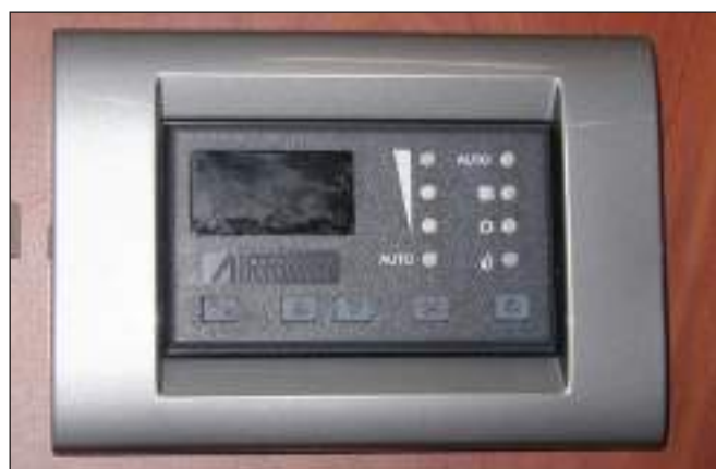
Typical Air Conditioner Control Panel
