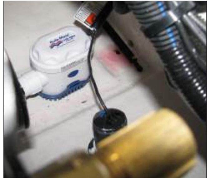
Aft Automatic Bilge Pump 214SS/218SS/234SS/238SS/268SS/288SS
