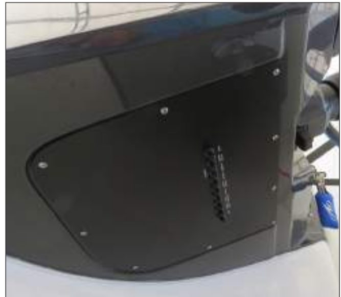
Helm Circuit Breaker Panel
