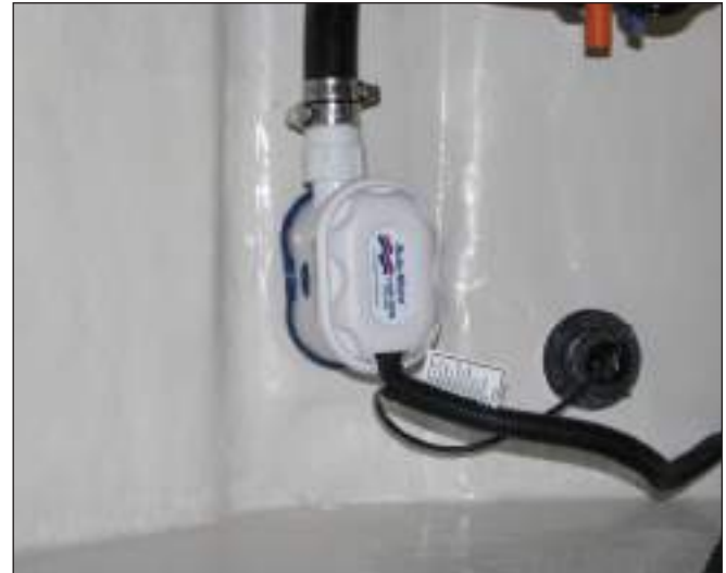
Typical Automatic Bilge Pump
