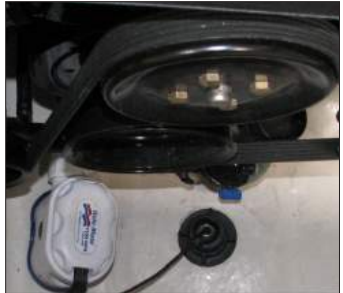
Typical Bilge Pump with Automatic Float Switch
