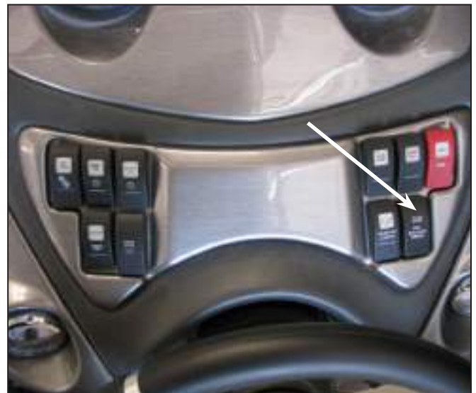
Ballast Tank Pump Control Switch
