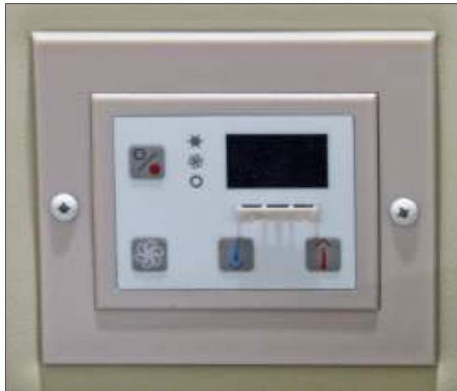
Typical Air Conditioner Control Panel
