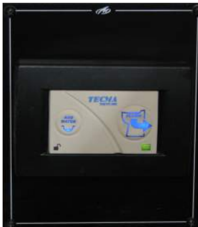
Head Compartment Toilet Control Panel
