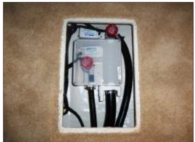
Typical Forward Bilge Pump, Automatic Switch & Drain Sump Pump
