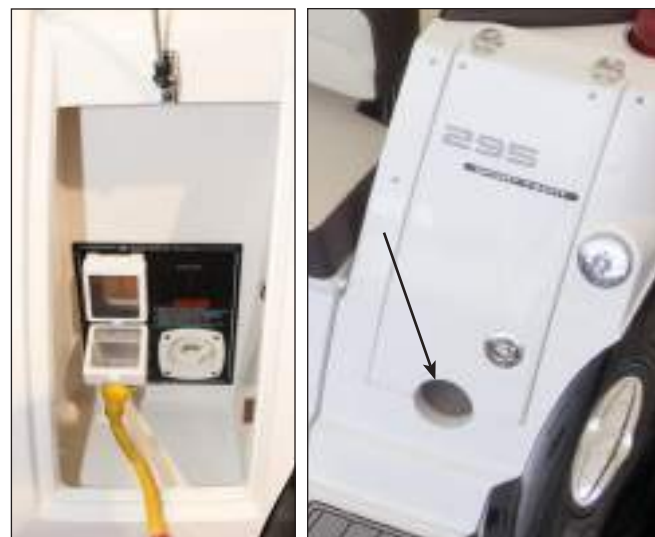
Shore Inlet Connection Compartment & Door With Cutout for Cables & Hoses
