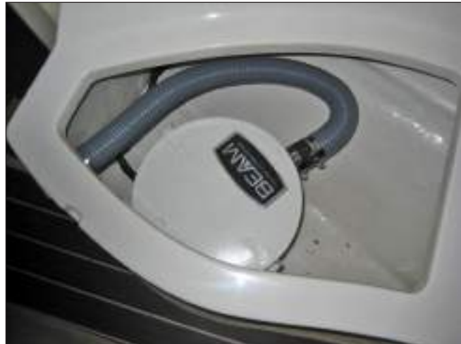
Typical Central Vacuum
