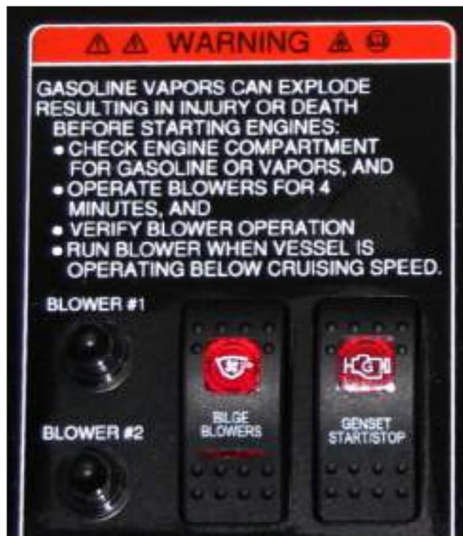
Generator Remote Control Panel in Cabin
