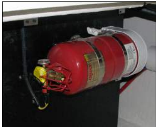
Automatic Fire Extinguishing System In The Engine Compartment
