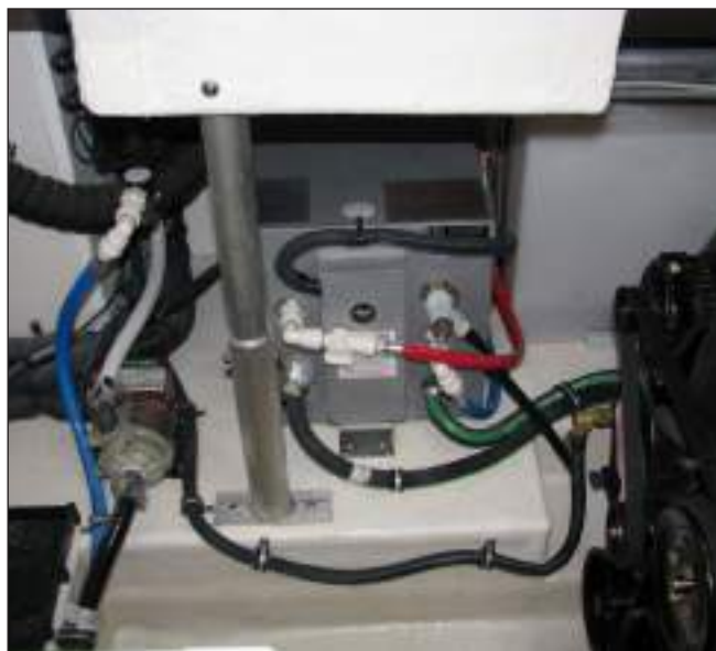
315SY Water Heater In Engine Compartment
