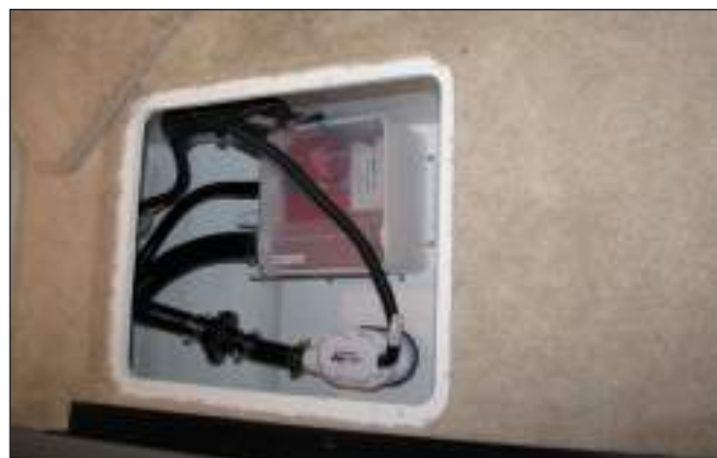
275/295SY Mid Berth Bilge Access Hatch
