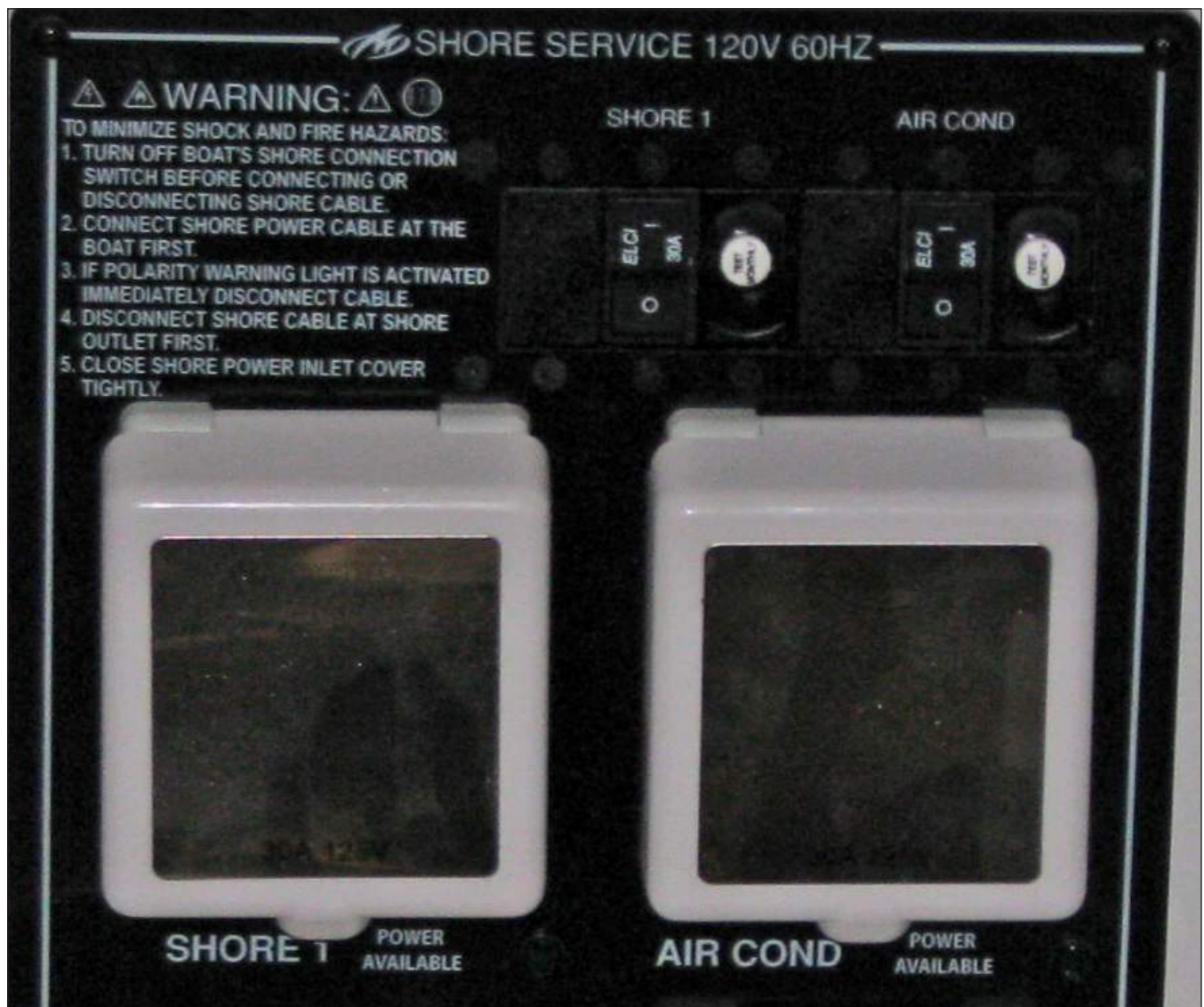
315SY Inlet Panel With Air Conditioning Option - ELCI Circuit Interrupter/Circuit Breakers
