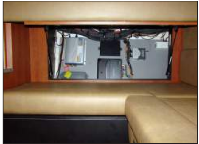
Equipment Locker and Remote Electronics, Inverter, Stereo Amplifier and Components
