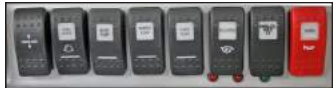
Helm Switch Panel - Starboard Side
