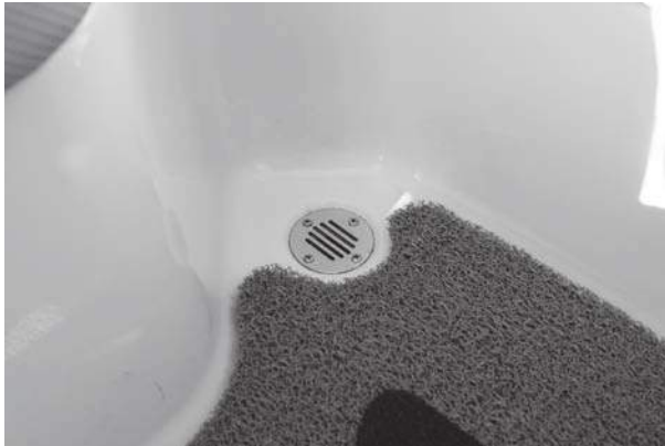
Figure B39: Liner Drain
