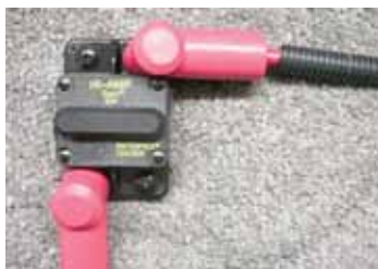
Figure 4-8. Main Circuit Breaker
