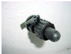
Lever on the aerator fitting is closed
