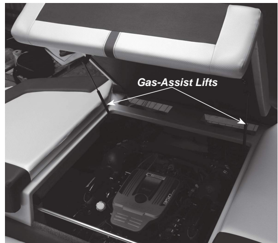
Figure N17: Raised Center Sundeck - Engine Compartment Access
