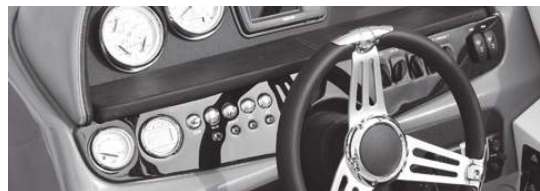
Figure Q4: Helm Switch Panel
