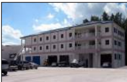
Valhalla Service Center, South Florida
