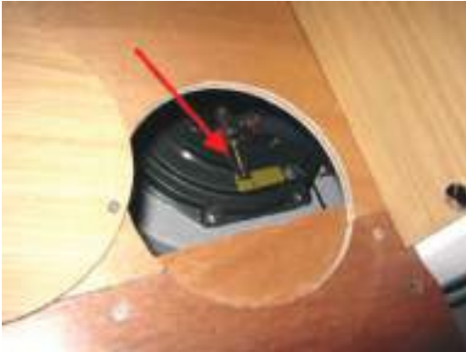
Access: Starboard aft cabin
