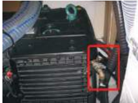
Supply valve - Water heater / Cooling system - Engine
