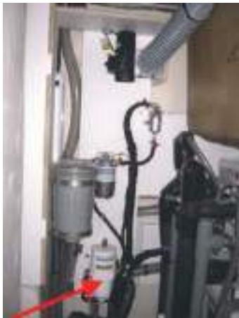
Access: Engine compartment
