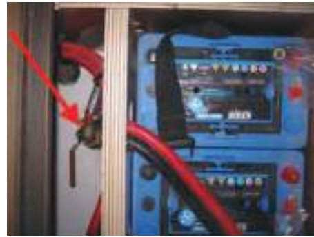
Sea water intake Access: Passageway - Galley
