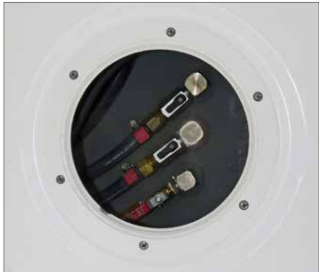
Typical Fuel Withdrawal Valves
