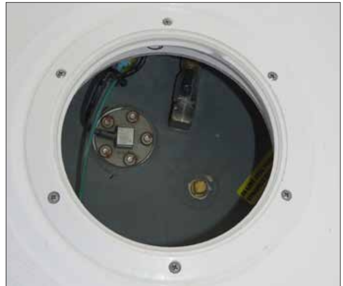
Fuel Gauge Sender & Withdrawal Valve
