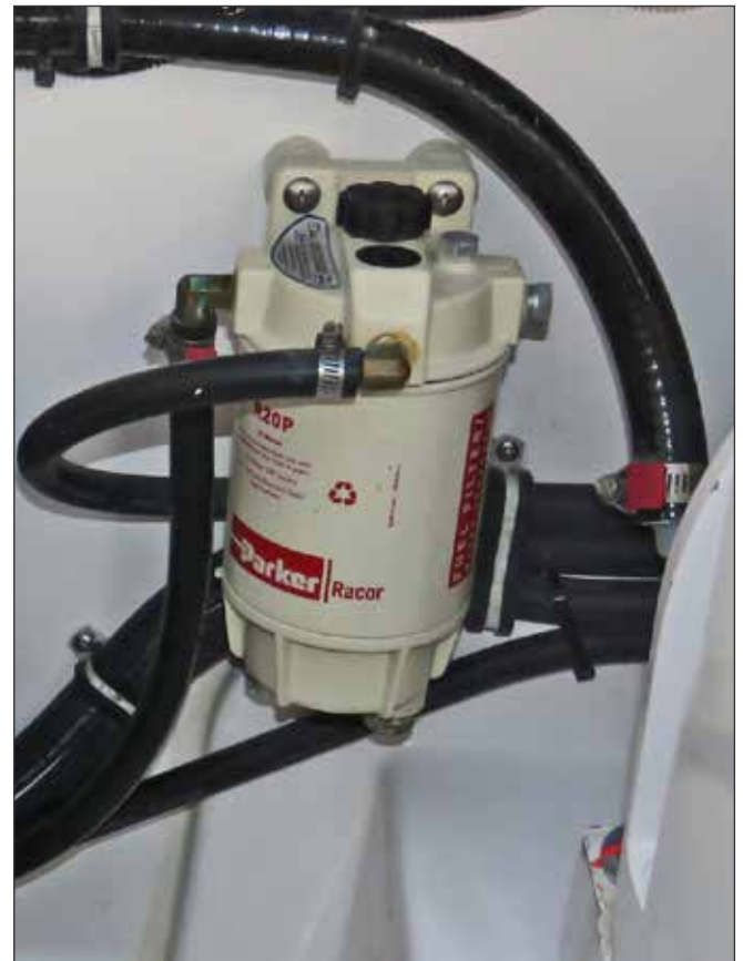
Generator Water Separator Fuel Filter
