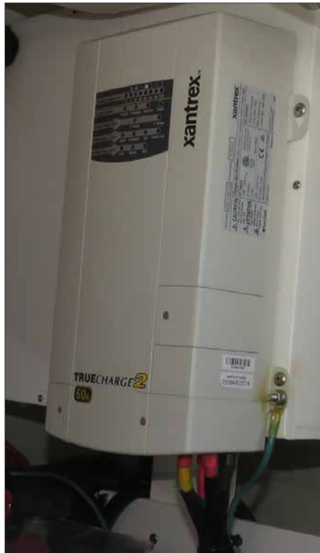
Typical Battery Charger
