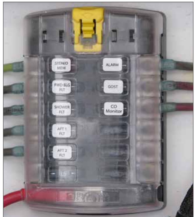
Continuous Power Fuse Panel
