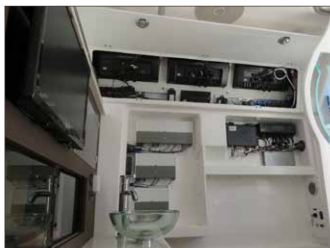
Electronics Access in Rear Cabin Bulkhead
