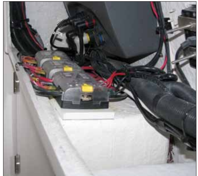
Electronics and Accessory Fuse Panels Behind Helm
