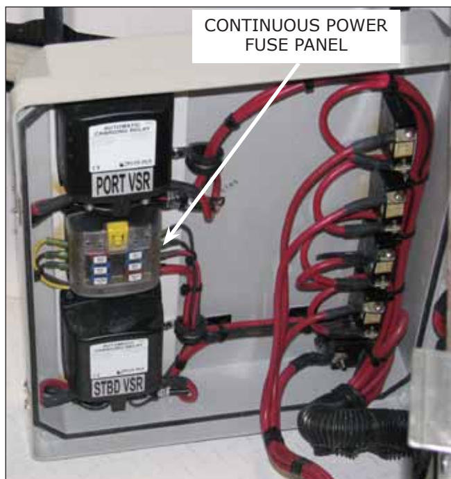
Main Circuit Breakers and Continuos Power Fuse Panel
