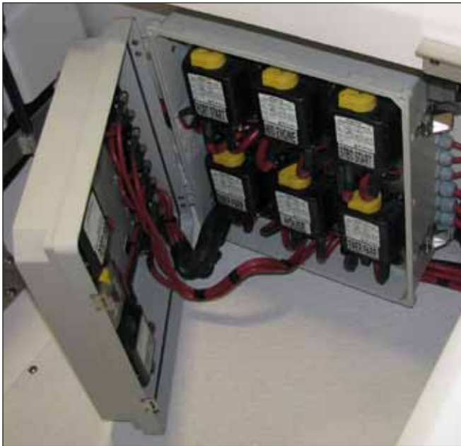
Battery Switches, Emergency Parallel Switches, PT & STBD Voltage Sensitive Relays, Main Circuit Breakers and Continuous Power Fuse Panel
