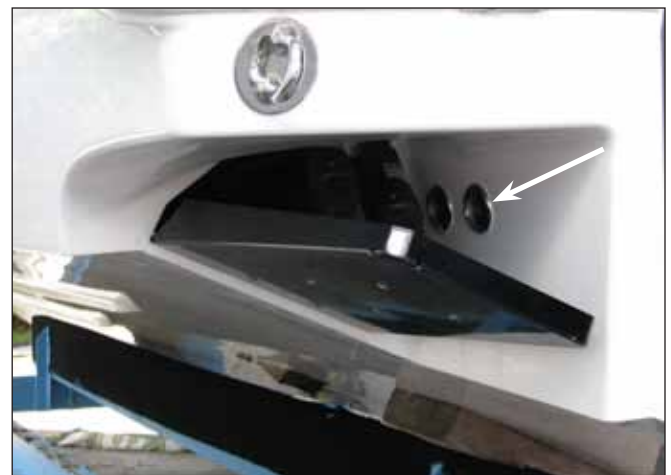
Scupper Drain Thru-hull Fittings
