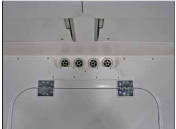
Typical Scupper Drains and Drain Rail
