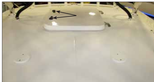
Upper Station Access Hatch Note exterior Access Hatch Cam Latch Levers
