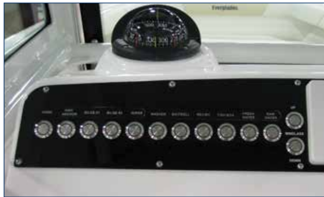
Port Side Helm Switches
