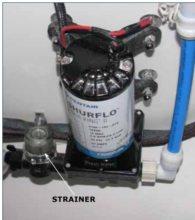
Fresh Water Pump & Strainer
