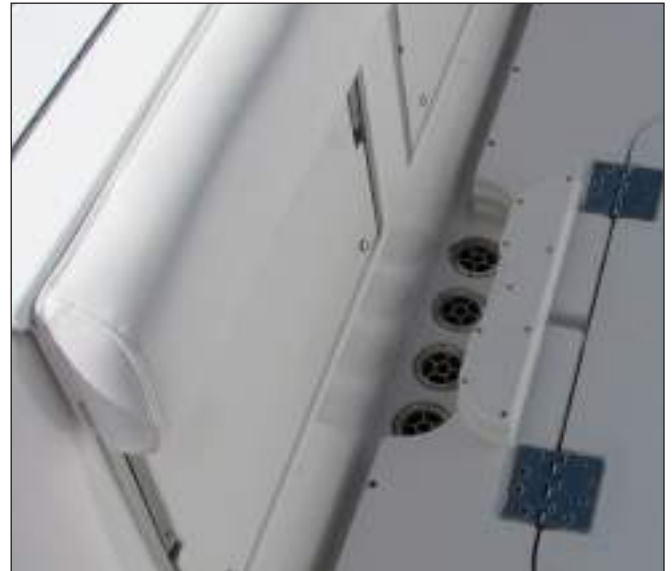
Typical Scupper Drains and Drain Rail
