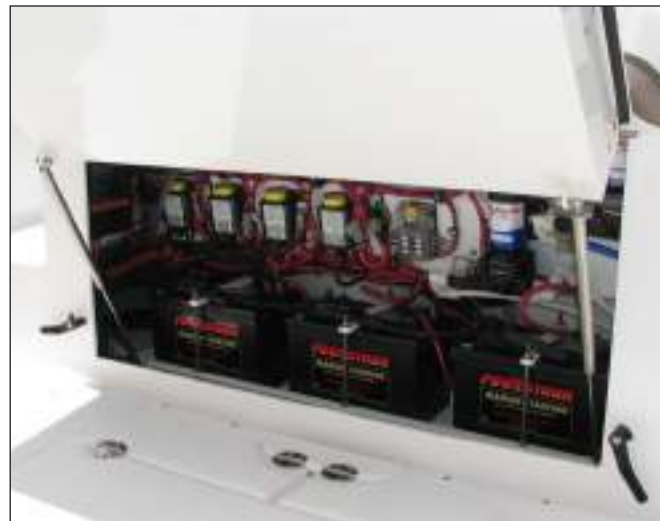
255/275/295 Center Console System Compartment and Batteries
