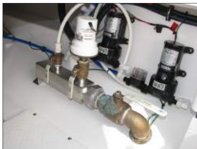
325 Center Console Seawater Supply Manifold and Seacocks Baitwell Supply Pump and Raw Water Pressure Pump
