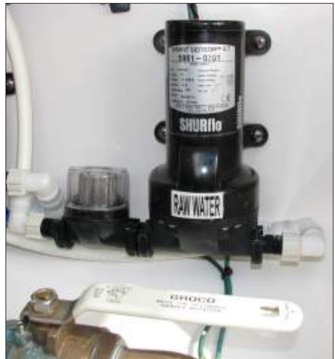
325 Center Console Fresh Water Pump and Strainer
