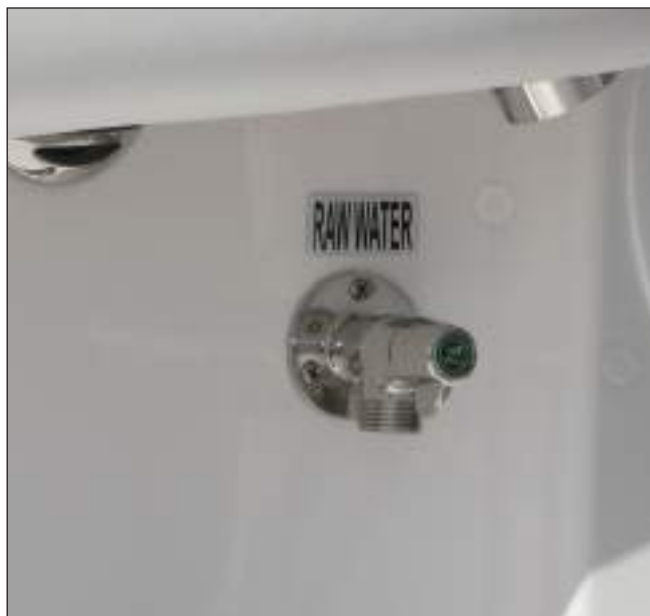
Typical Washdown Hose Connection
