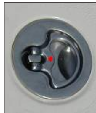
Twist Latch Unlatched Red Dot Showing
