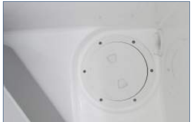
Forward Bilge Access Hatch
