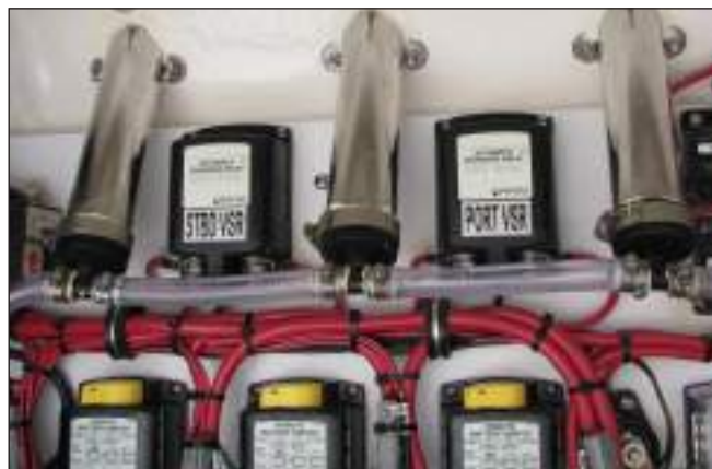
Voltage Sensitive Relays 255/275/295 Models
