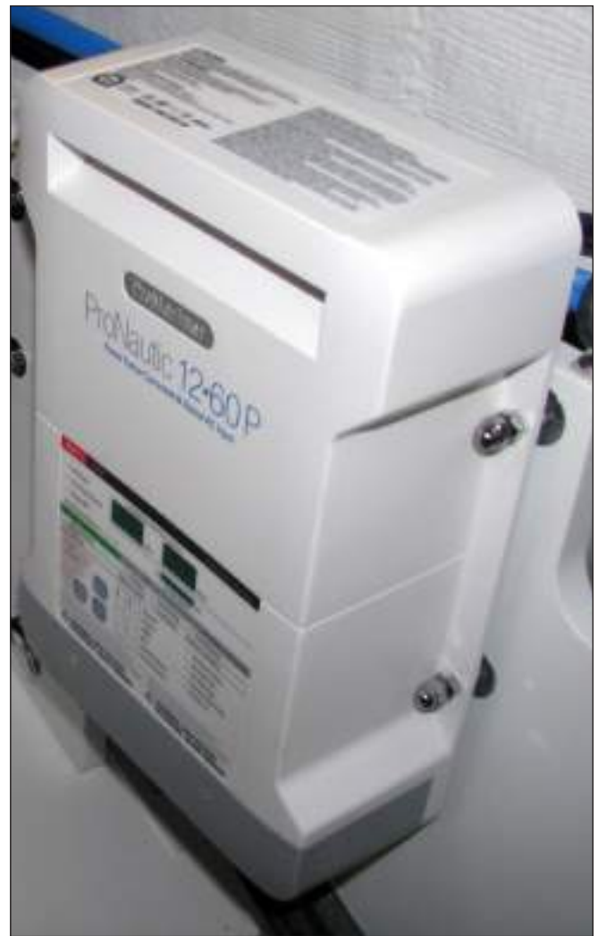
Typical Battery Charger
