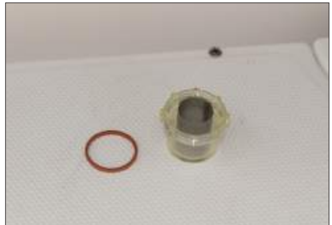
Typical Raw Water Pump Strainer Removed for Cleaning
