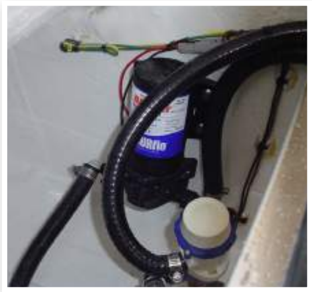
Raw Water Pump
