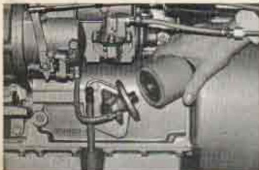
Fig. 14. Replacing lubricating oil filter
