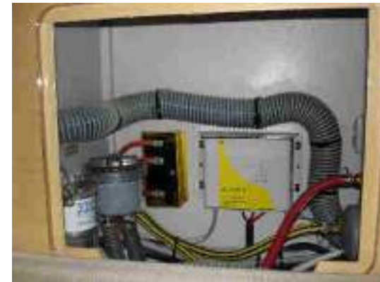
Charger to port in engine compartment on cabin side
